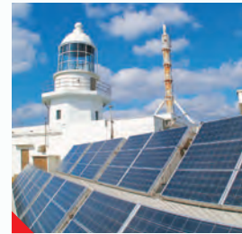
▼1966 PV panels power Ogami Lighthouse, Japan
