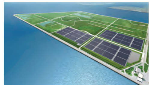
Sakai Solar Power Station
